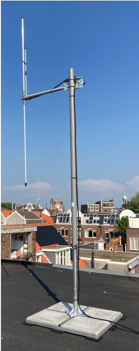
The 4m Half Wave Dipole with GM. Installed on a new tile frame with a mast of 120cm. On top of it you see a
