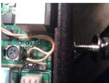
Punchdown wire soldered to open SMD fuse
