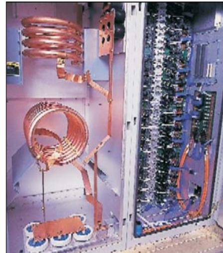
**Figure 16 . Output section of a 50-kW AM broadcast transmitter.**
