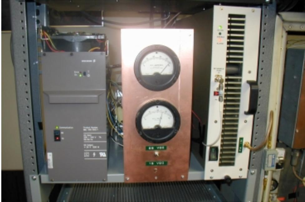
**Figure 7** Front view of Spectrian amplifier tray, shown keyed at full power out.
