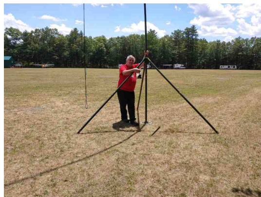
Joe KA1GDQ holding mast while guy wires are attached.
