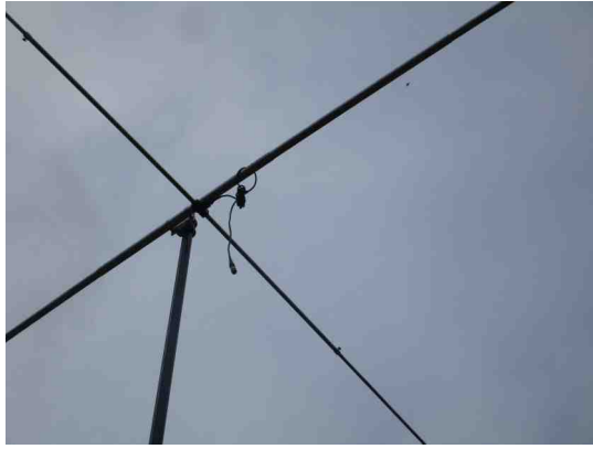
Beam up on the mast, but missed one step. Failed to connect the coax.
