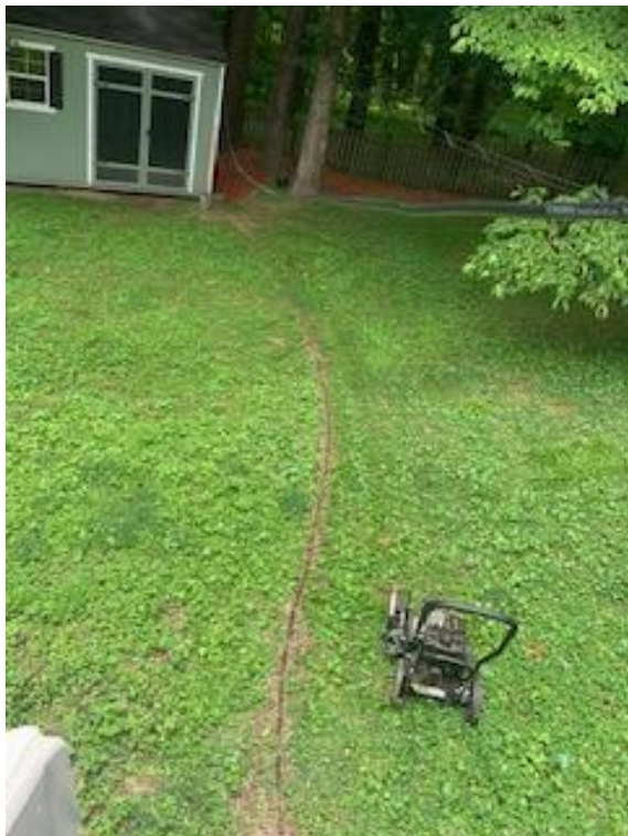
Picture 3 – The buried feed line and ground wire
