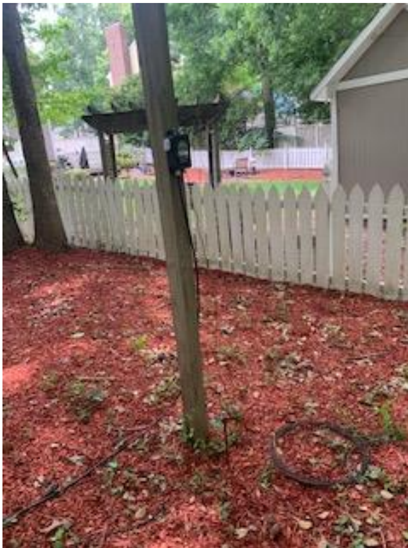
Picture 2 – The antenna mounted on the fence post
