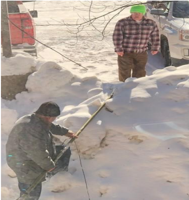
Greg and Fred installing HQ antennas.
