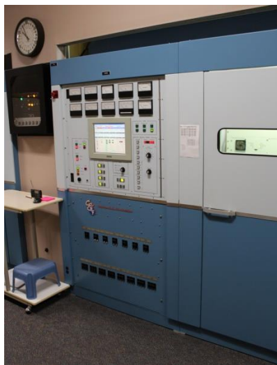
One of the two 100 KW transmitters.
