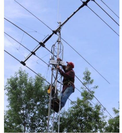
Greg, KI8AF, on my tower. Note that he is always properly belted in and that his tool bag is on a separate line.
