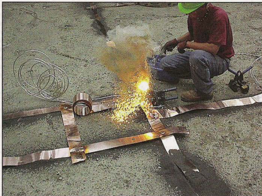
A worker "Cadwelding" (see text) #2 solid copper wire with 4-inch-wide flat copper strap. The dark material around the copper strap is Harger "ground enhancement."
