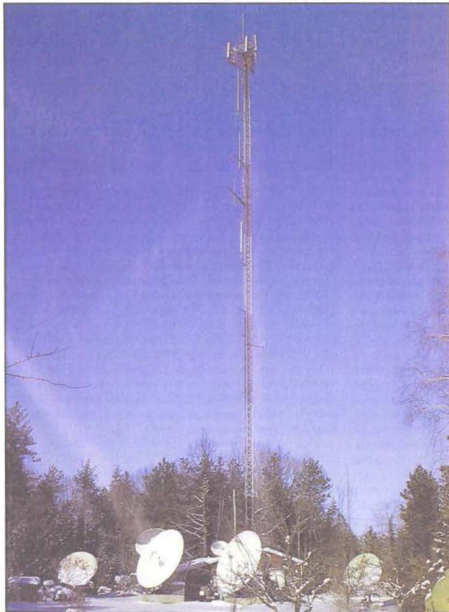
Or think tall...A PiRod 200-foot commercial tower recycled to ham radio use when the cable company went to fiber optics. This photo also shows some satellite dish antennas.
