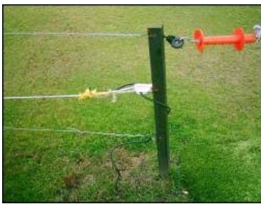
Above: The power leads coming up out of the ground to link the wires together – note the inadequate use of insulation tape!
