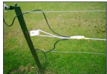
Above: The power leads coming up out of the ground to link the wires together – note the inadequate use of insulation tape!
