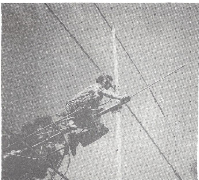
A missionary doctor on his day off! Dr. David Stevens, 5Z4DL, Tenwek Hospital, Kenya. Installing a lightning rod after securing the beam. The 60-foot tower was pulled up by a Bob Cat.
