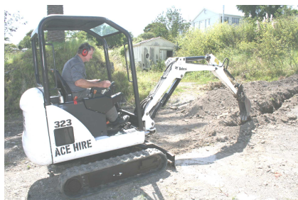
Digging the trench for the phone line
