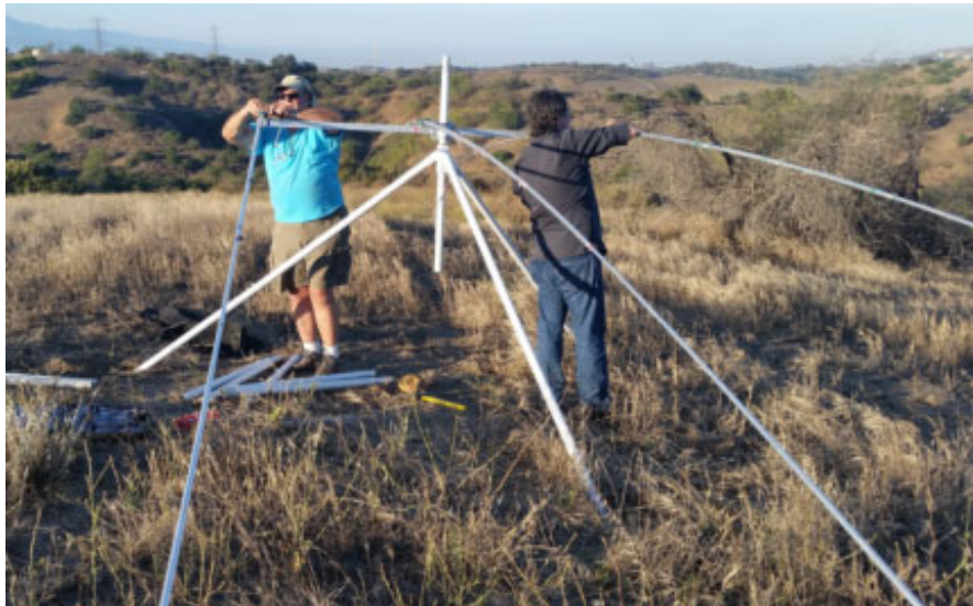
Bob, AA6PW (L), Wes, W3SE/ZL3TE (R) Assemble the 20 Meter 3 Ele Log Periodic ( Engineering Prototype )
