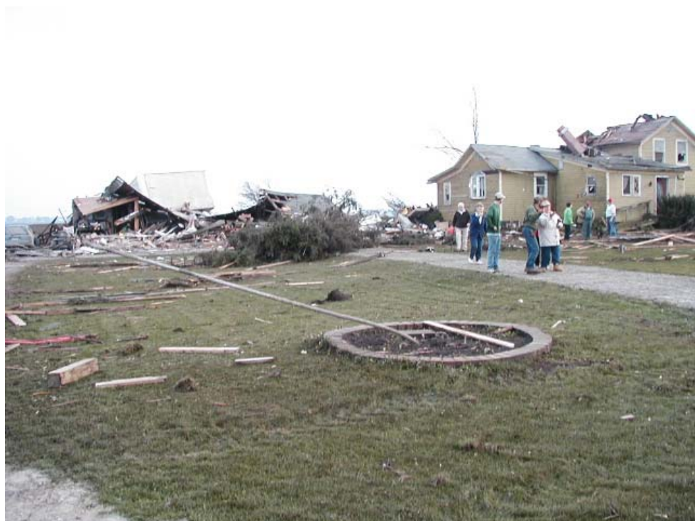
Structure Damaged by Tornado in Putnam County
