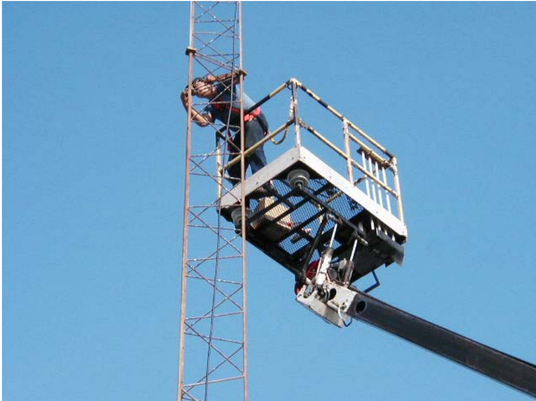
Worker Dismantles “New” SRRC Tower
