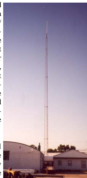
Tower at Otter Creek Twp Garage
