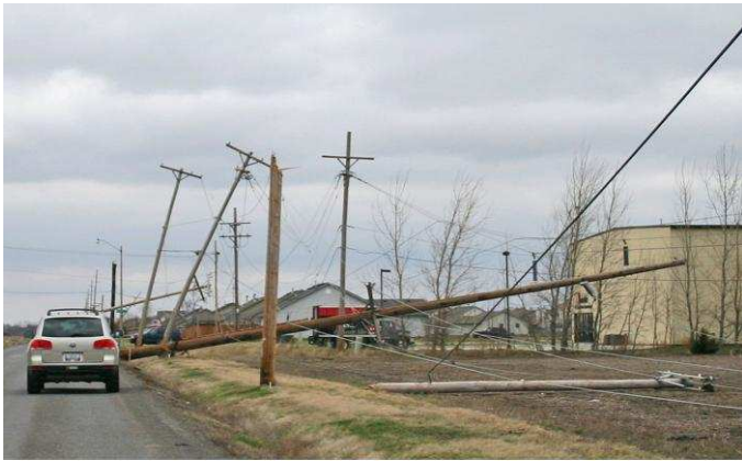
POWER POLES DOWN ON ARCHER ELEVATOR ROAD
