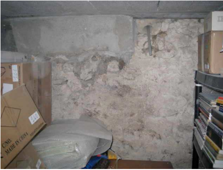
Basement side with new hole, not too bad with no point of reference for the hole, conduit in place.
