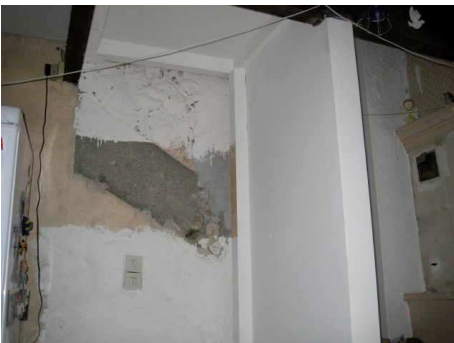
Outside kitchen wall after opening it up.
