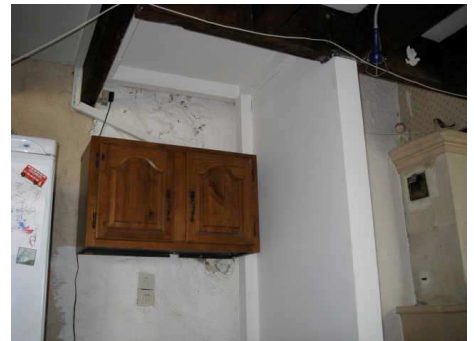
After interior hole with cabinet back in place
