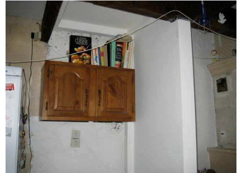
Before interior hole
