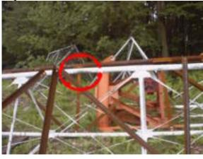
You can see the tower legs were bent by looking down the tower. Look down the top rail of the tower and you will see that it is out of alignment by about 4 inches. The pictures were taken from the ground. The small plane was going north from Clarksburg, where he
