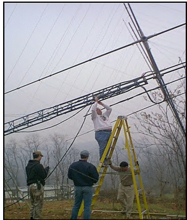
Raising the K3JT Cubical Quad.
