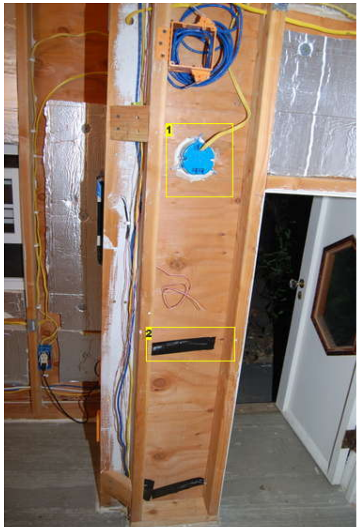
Image Notes 1. Porch light 2. 12V Wiring for Doorbell
