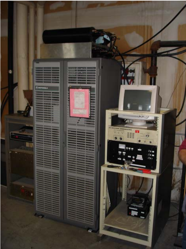
The new Micor cabinet (Left) Old Equipment Rack (Right) with Monitor, Spec- trum Repeater, Voter and Packet Station
