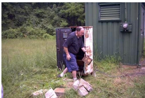
Dick removes equipment from old Linvale cabinet
