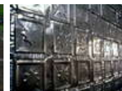
Press Aluminum Cans into Ceiling and Wall Tiles by robbtoberfest
