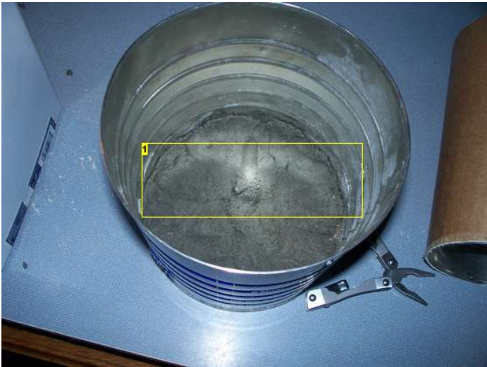
Image Notes 1. fill bottom with Quickrete up to the hole. pack well
