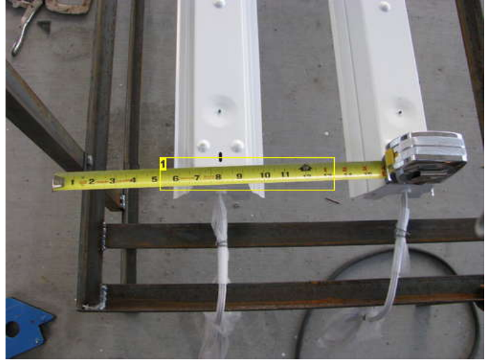
Image Notes 1. Measuring front to back offset.
