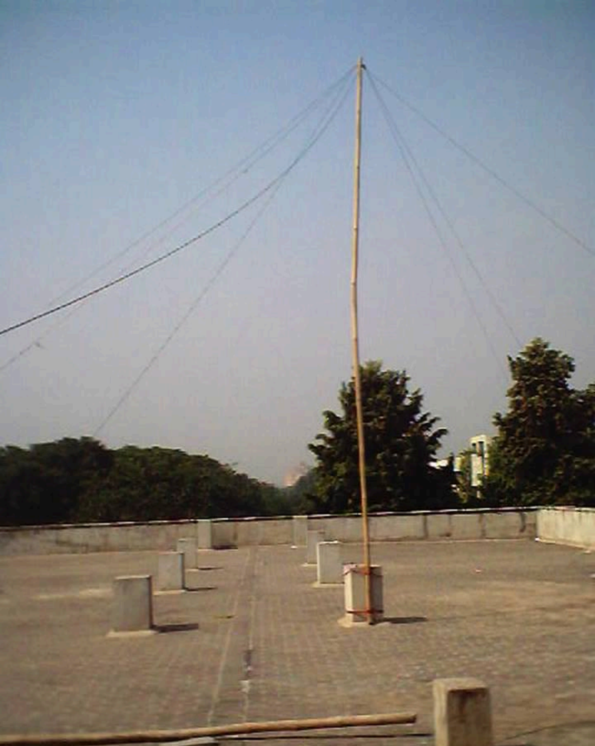
Antenna Installation at a demo site
