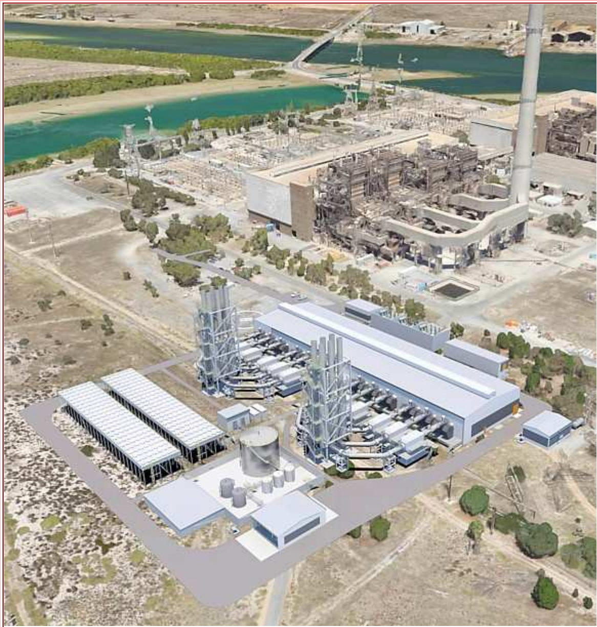
Torrens Island Power Station A is shown above with an artist impression of the Barker Inlet Station below
