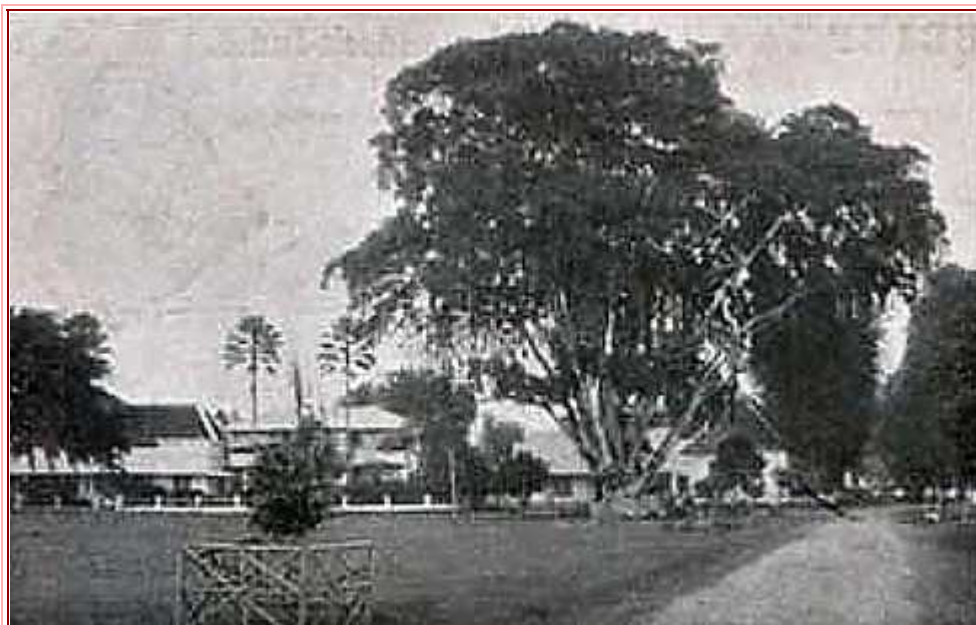
Banjowangie Cable Station, Java
