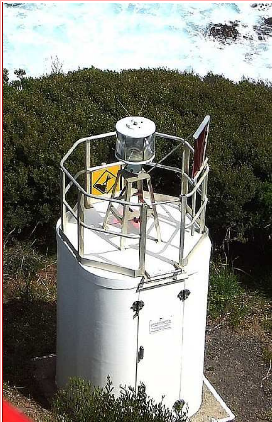
This solar powered beacon replaced the light mechanism of the original tower in 1994
