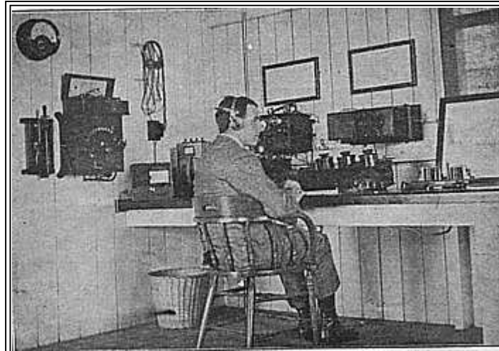
Figure 19 Interior of Station at Suva, Fiji Islands. (Ref. 1)
