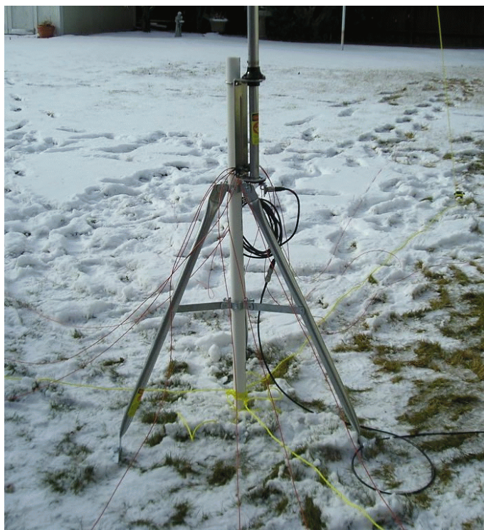
The PVC pipe is installed inside the tripod, the antenna base is clamped to the PVC, and the radials fall to the ground.
