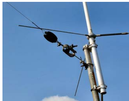
right: the other attach point at the V2000 mast, including the turnbuckle. With the turnbuckle wound up this way, it shows how optimally the antenna length has been used.
