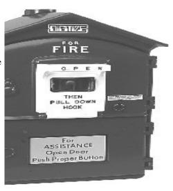
Telegraph systems? Well, a couple of things. First, box alarms are probably the only 19th century technology that is still in everyday use. It's in use because, simply, it works. No VLSI chips, no routers, no ISO 7 layer model. Just a clockwork wheel that breaks a circuit. Here's what happens when you pull the box to report a fire
