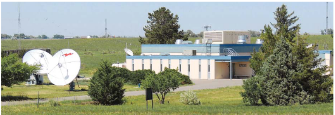
Timing, signal-generation, and transmitting equipment can be found in the radio station's main building.
