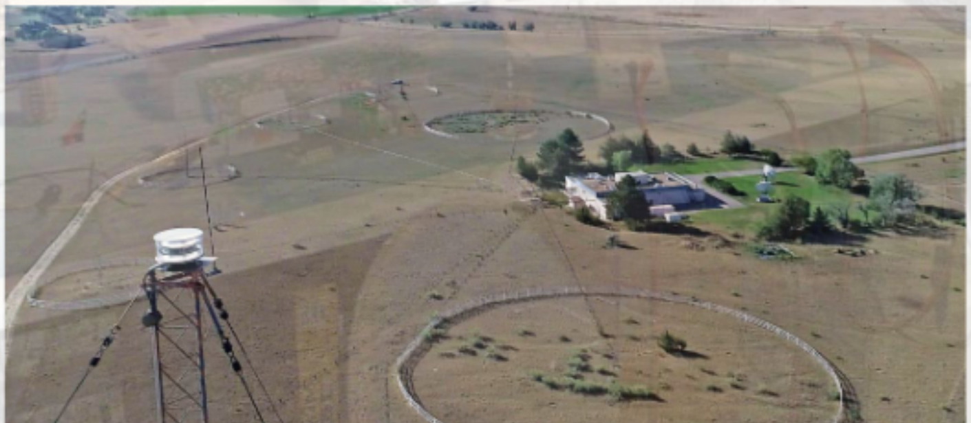
An aerial view of WWV. The station broadcasts six frequencies with their own antennas, which are all surrounded by a white fence. The lowest frequency has the tallest antenna, and it requires a flashing strobe to be visible to passing aircraft.
