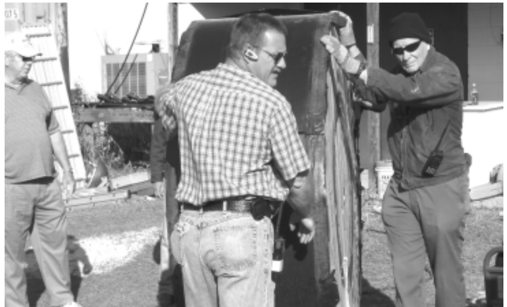
Barry (WB5WB), Ray Luke, chief engineer for WXXV-TV, and Tom (W4WLF) prepare to move a spool of heliax cable to prepare it for going up the 1,478 foot WXXV-TV tower
