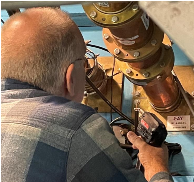
John prepares a replacement coax connector.
