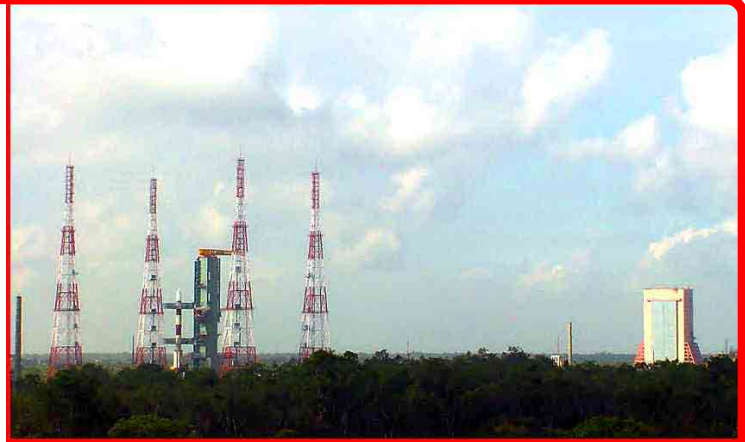
The Satish Dhawan Space Centre (SDSC) in Sriharikota. 360+ foot tall lightning protection towers dwarf the 200 ft. PSLV-C6 launch vehicle. The vehicle assembly building is to the right.
