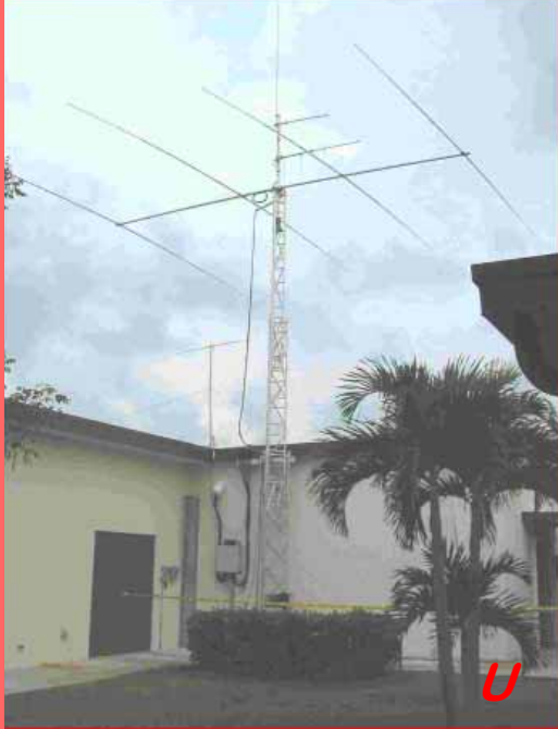
U -Four element 20m beam at 33 feet provided punch on the most congested band. V -Supporting the legs of the 309 foot Vee Beam were 40 foot towers. W -Murphy strikes... steel pipe at top bent like a toothpick during the raising of the west leg of the Vee.
