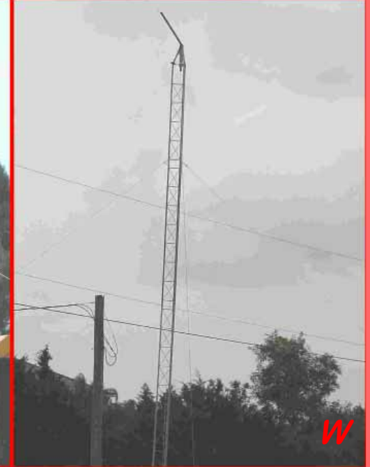
U -Four element 20m beam at 33 feet provided punch on the most congested band. V -Supporting the legs of the 309 foot Vee Beam were 40 foot towers. W -Murphy strikes... steel pipe at top bent like a toothpick during the raising of the west leg of the Vee.
