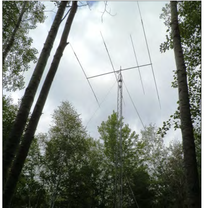
The rebuilt A4 on a 56-ft Rohn 25 tower, which is located 350 ft away, back in the woods.
