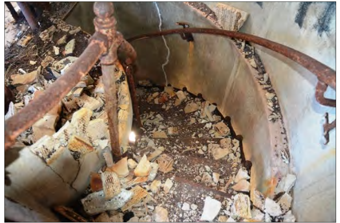
Deteriorating condition of lighthouse staircase. The bottom of the lighthouse was worse, with several inches of debris, plus trash left behind over the years.
