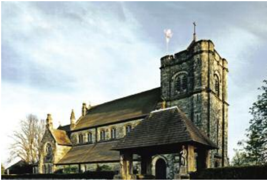
St Leonard's Church, Turners Hill, West Sussex. The flagpole atop the tower conceals the antenna for GB7MH.
