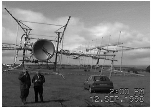
The assembled array ready for erection
