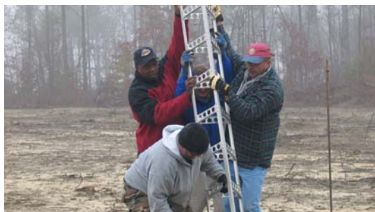
Quint, and Rich (KI4EUM) steady the tower as Barry (W3AFH) prepares to insert the pin
