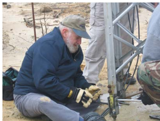
Sonny (K4WYS) makes final adjustments on the 40' Rohn BX tower
