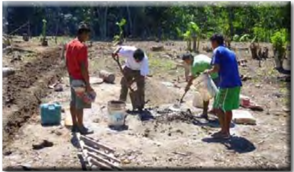
Mixing cement by hand.
