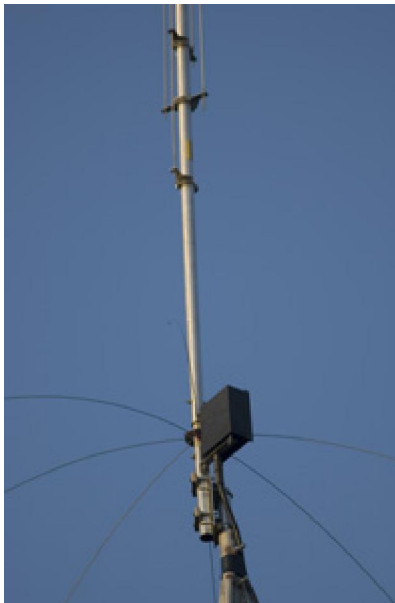
Matching network and base of stubs
