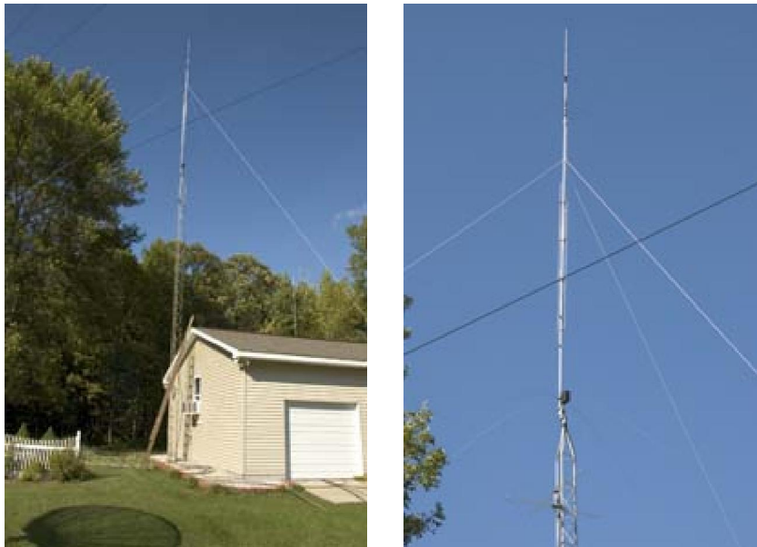
Two views of the AV-640 and tower
