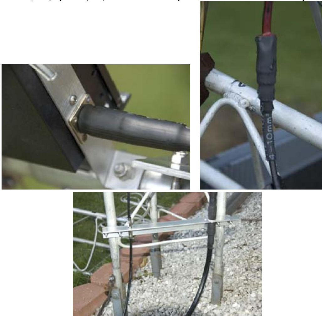
The new Lexan (TM) spacer (left) and the weatherproofed connection for the top loading (right)
